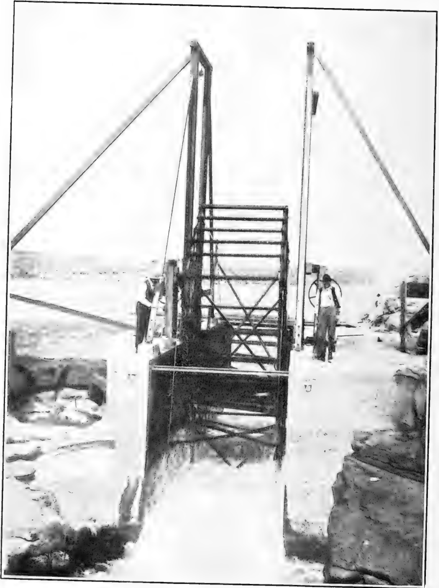
FIG. 25.—A COLUMBIA RIVER STATIONARY FISH WHEEL
